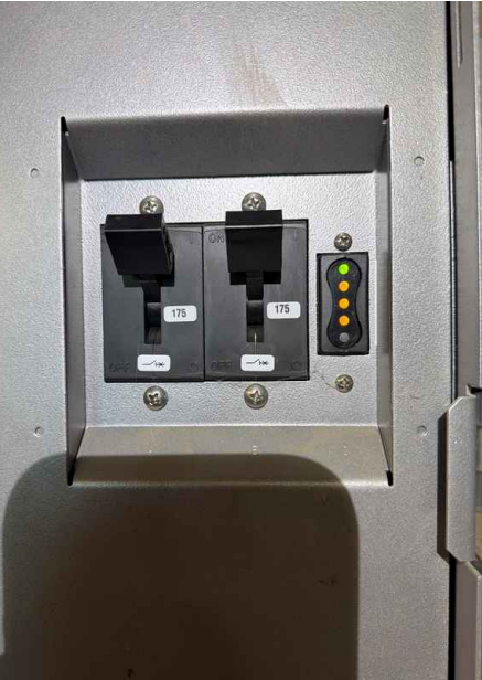
Main & Subpanels, Service & Grounding, Main Overcurrent Device: Panel Capacity - main 175 AMP
